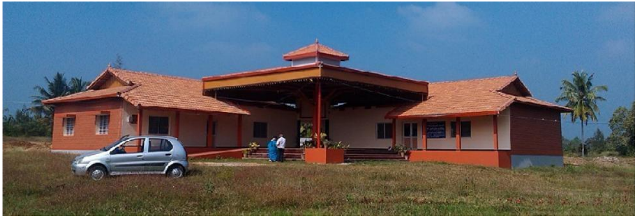
a. 1 st Phase of Sharanya Hospice Care Center Building which is ready for In House Palliative Care for Terminally Ill Patients of Cancer.
